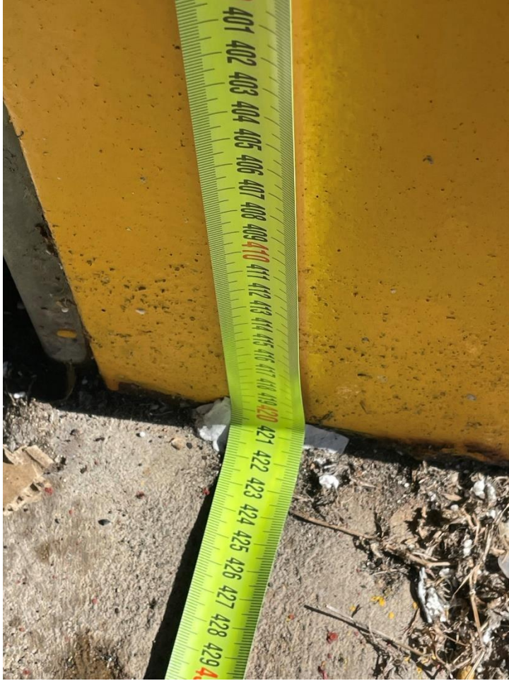
Door opening western side
