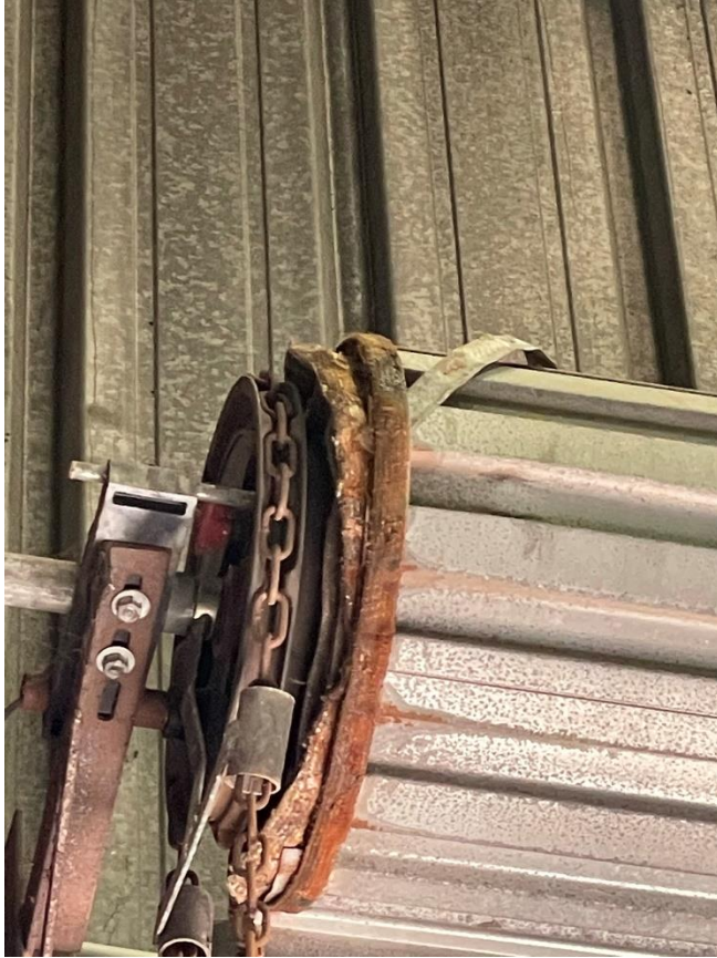
Nylofelt pulling off western side; motor is attached to this side
