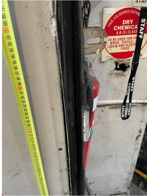
Damaged guide
