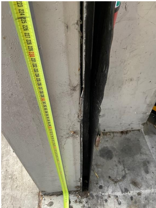
Damaged guides
