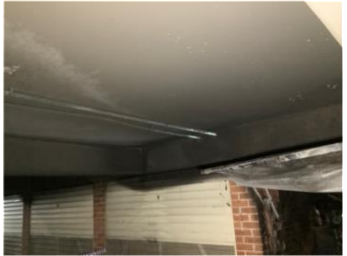
overview carpark area and existing services
