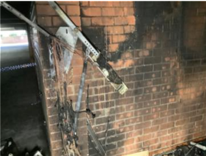
cause of fire advised as overloaded power
