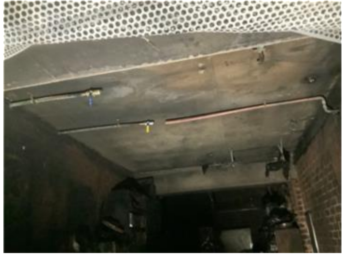
disconnected/made safe services in unit 7 garage
