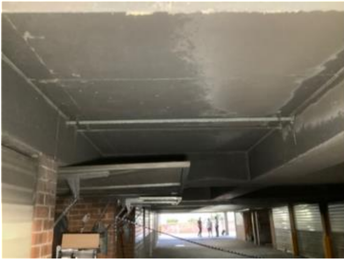
overview carpark area and existing services
