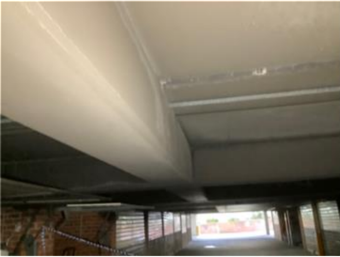
overview carpark area and existing services
