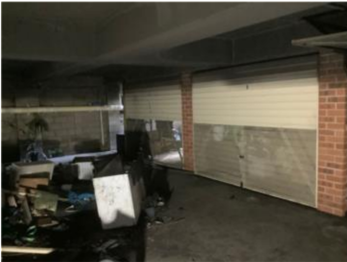
overview - unit 8 garages opposite unit 7 garages
